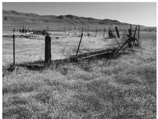
A now-abandoned corral made from the remains of a transcontinental railroad trestle, photographed in 2017. The corral was built during the 1980s, an act that, while destructive in nature, showed the need for wood in this barren environment. Photo by Glenn Stelter.
