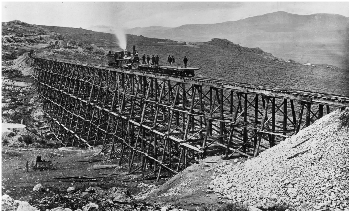
A wooden trestle spanning a 450-foot-wide cut on the Union Pacific Railroad line east of Promontory.
